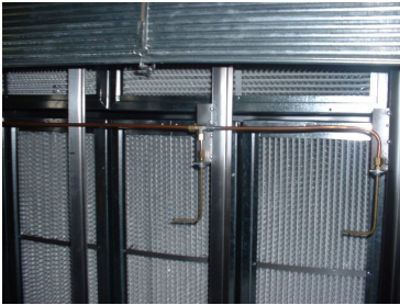
Box Filter probes as viewed from discharge
