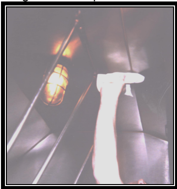
Wipe Interior of Hood
